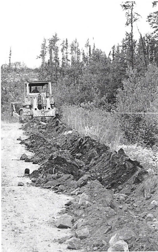
Fig. 3. Fiat HD-21 tractor 'ripping' road with use of a V-plow.
